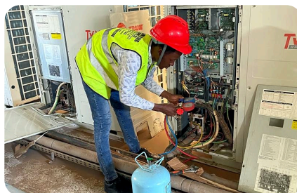
Air-conditioning servicing
