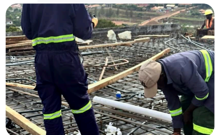
Electrical first-fix on a large slab
